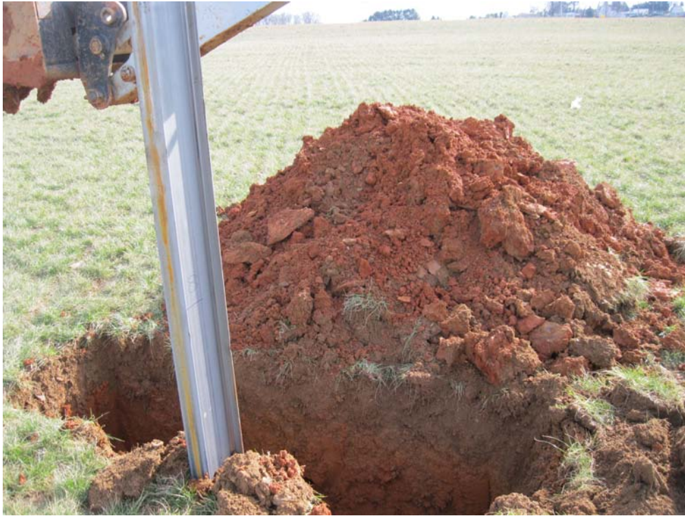
View of KTP18 excavation pit and soils pile.
